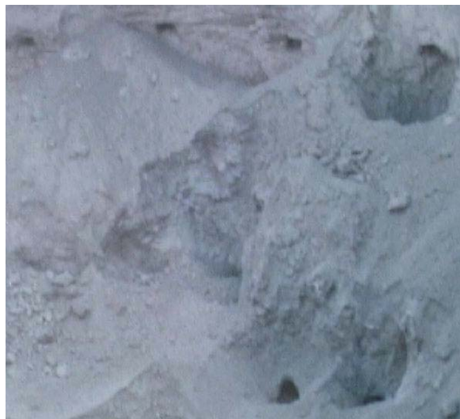
Ventilation openings into the De Beers' Koffiefontein mine's underground workings – in the pit among heaps of dusty and dangerous weathered kimberlite.
